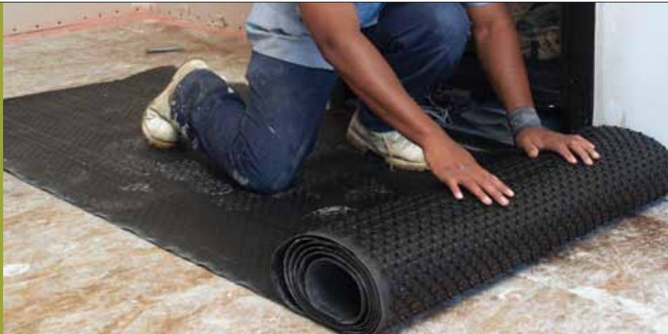
**A Connecticut contractor's flooring systems use LEVELROCK™ SRB™ sound reduction board and LEVELROCK™ SRM-25™ sound reduction mat to help builders and architects significantly reduce sound transmissions in various multi family projects.**
