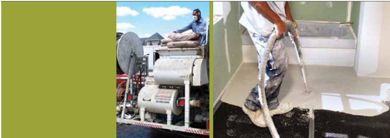
The first-floor living spaces of each building in Courtyard at Heritage Green sit over a parking garage and feature steel bar joists and a 3-inch concrete deck. The second and third floors have 18-inch wood floor trusses, a 3/4-inch tongue-and-groove subfloor and a 1-inch poured LEVELROCK 3500 floor underlayment installed over a 1/4-inch LEVELROCK sound mat system.
