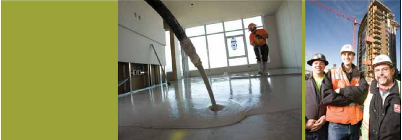
a precise amount of water is added to the underlayment/sand mixture and pumped up to the floor, where it is poured to meet the height of the grade pins. The material is then finished smoothly.
