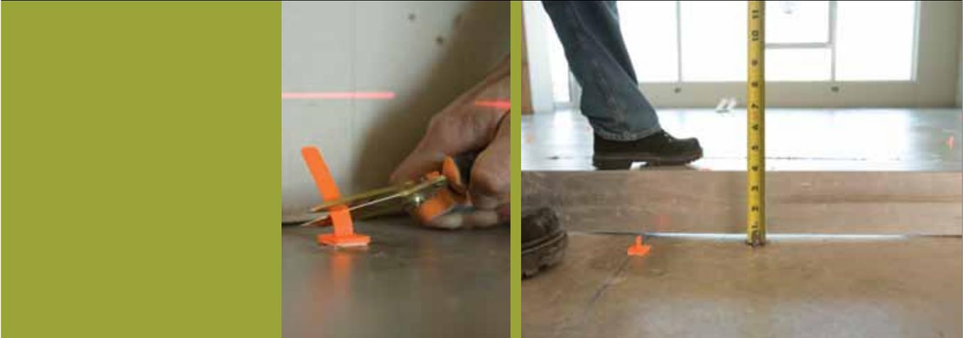
Knittel, a 30-year industry veteran of building big-city skyscrapers, says that's to be expected. However, to accommodate hardwood flooring, the decks had to be expertly leveled. Initially, Andersen Construction was leveling the subfloors on its own with a pre-sanded, bagged material - doing the work all by hand.
